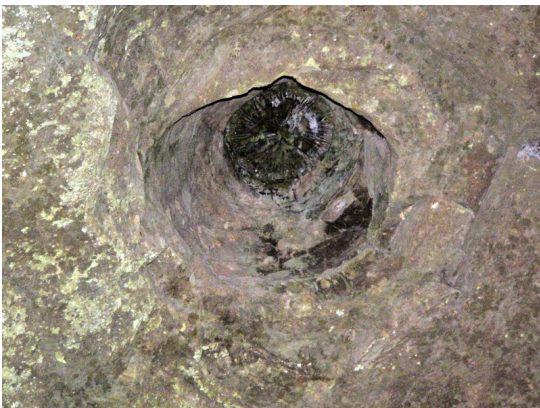
A buried tree in the ceiling of the North Falls Amphitheater
